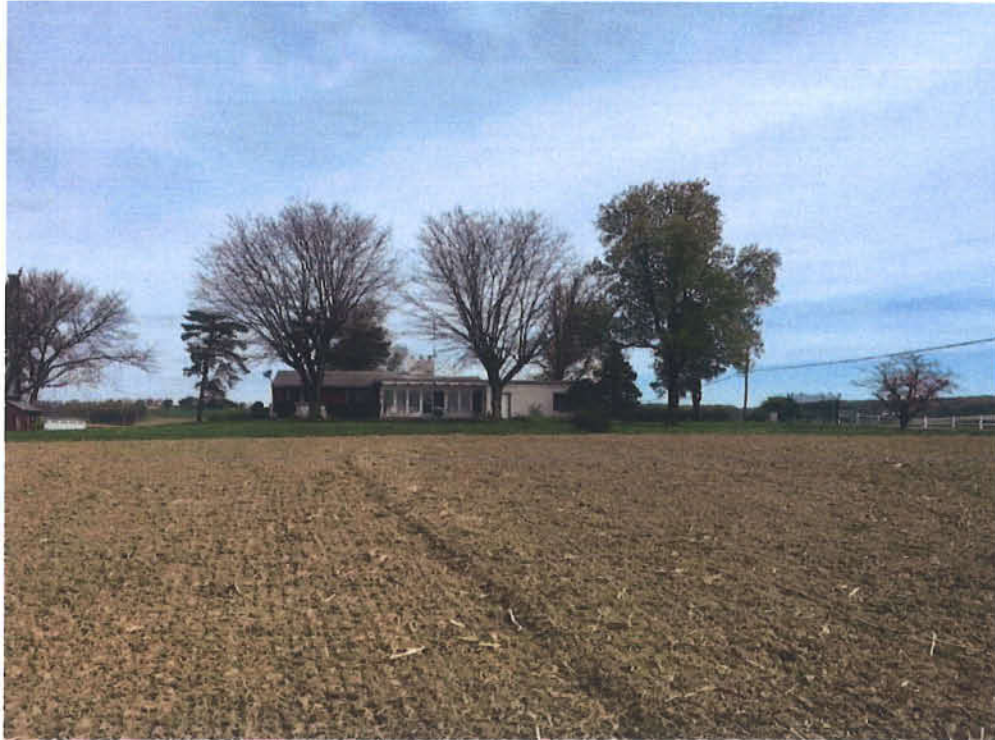
Photograph 3: Non-contributing farmhouse to the Richmond-Maxatawny Rural Historic District (Key# 204039) in the northeastern corner of project area.
